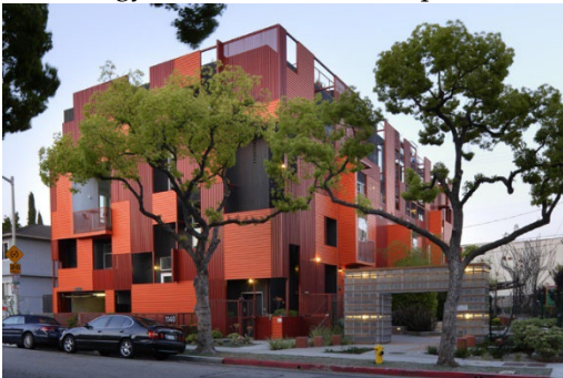
Figure 1a Ground floor, looking onto park
