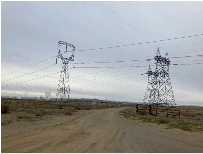
High Voltage Transmission Lines and Towers near Boardman, Oregon
