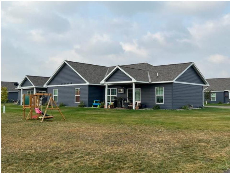
This is the backside and backyard of the home shown above.
