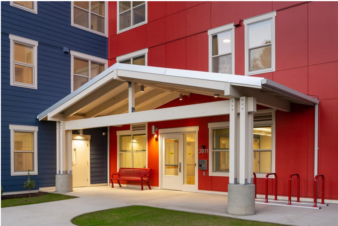
Arlington Drive Youth Campus in Tacoma, WA. Source: PCS Structural Solutions
