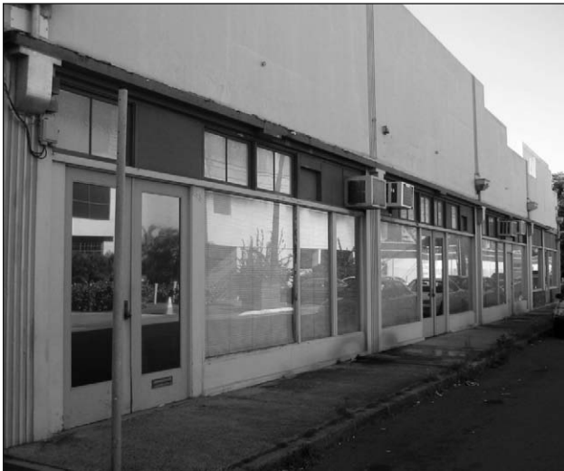
HOT box office, administrative office street frontage, before...
