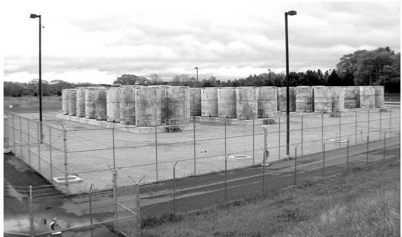
These 64 vertical concrete casks at Maine Yankee's ISFSI enclose sealed transportable storage casks filled with spent nuclear fuel.
