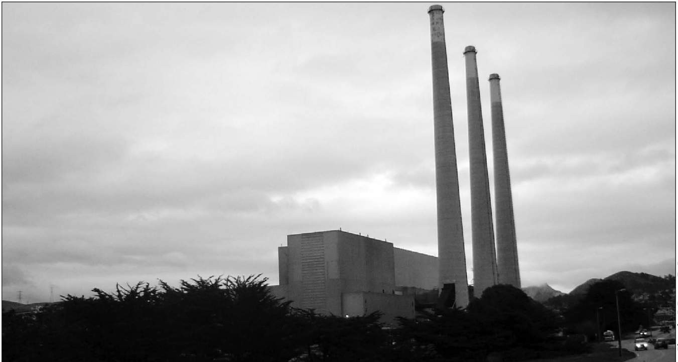
Traditional thermal power has long been generated by oil-, gas- or coal-fired plants. This one-time 1000-plus MW natural gas-fired plant has been relegated to use as a peaker 3 station on the California coast—its future may be backing up nearby solar projects in San Luis Obispo County.
